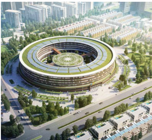
The EDGE-certified FPT Complex in Danang, Vietnam.
